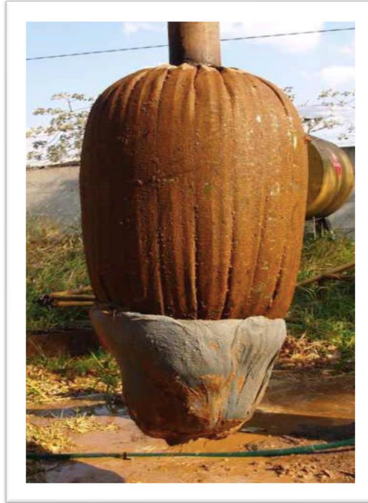
EXHUMED EB WITH POST- GROUTING
