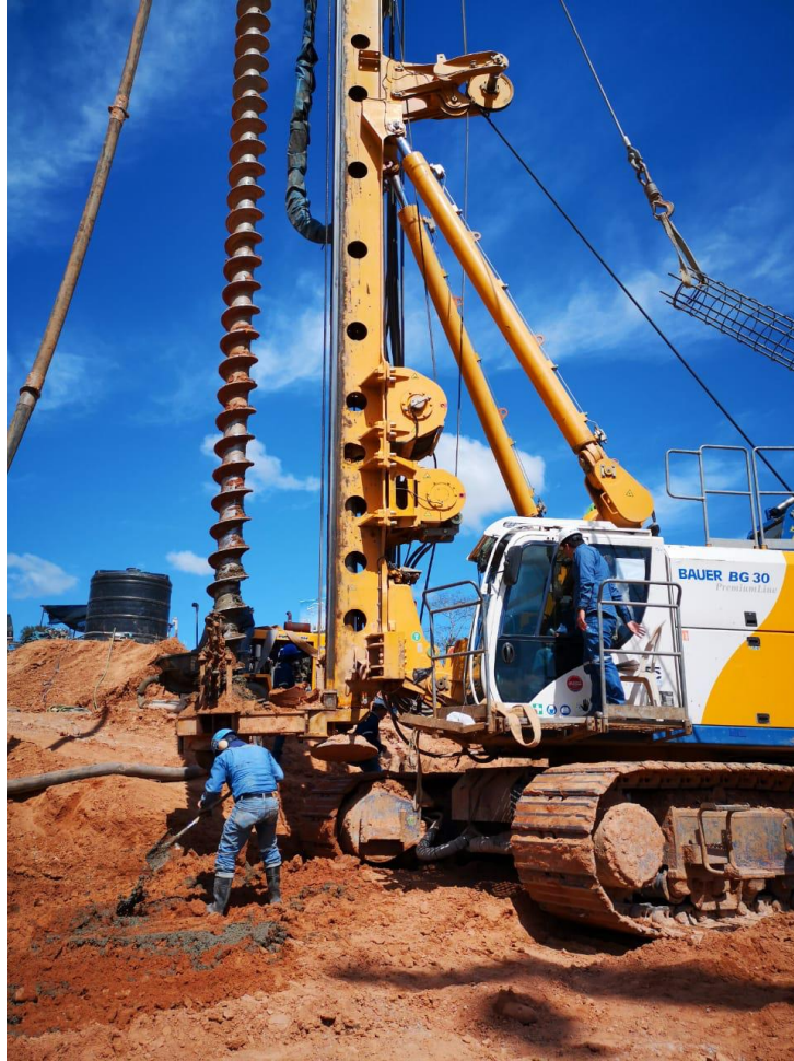
Partial Displacement Auger pile with EB achieves higher shaft resistance than regular CFA and high toe resistances.
