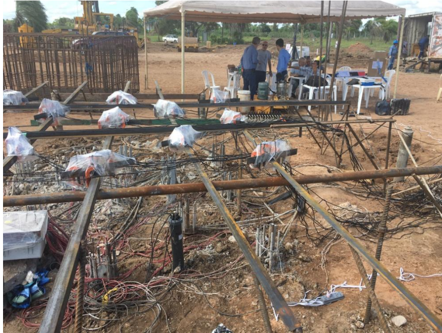
Fig. 7 Photo of frame for recording pile movements at Phase 1 test on Piles E2 - E14.
