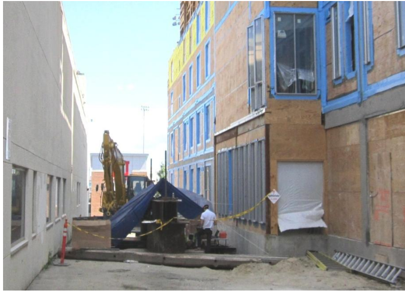
Figure 2. Photo of test site during ongoing static loading test
