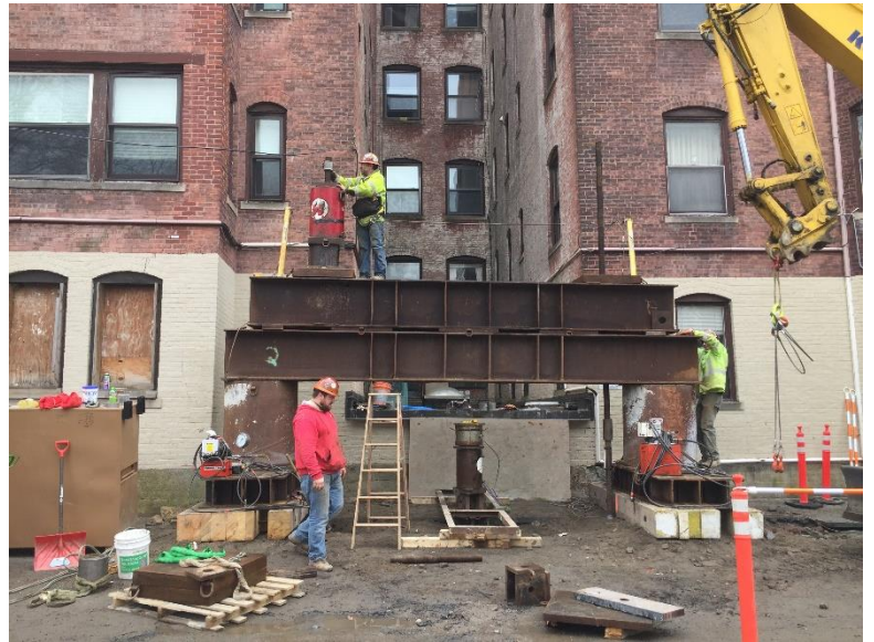
Photo 3: Test Frame Setup
