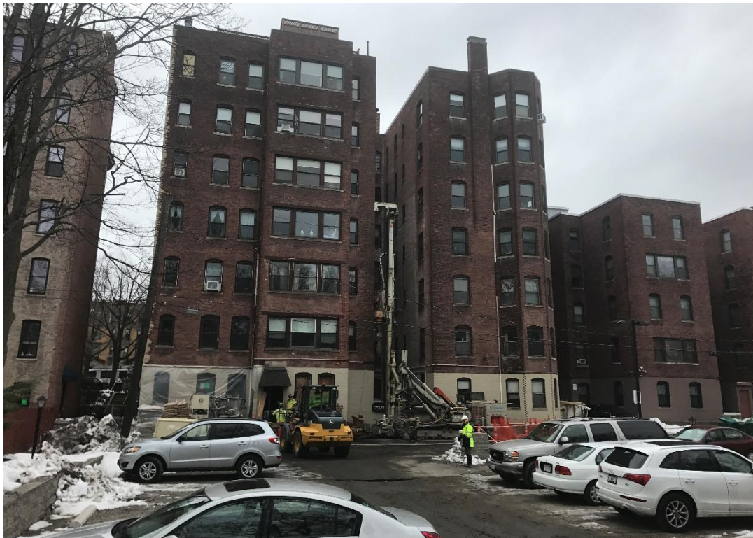
Photo 1: Drill the Test Pile on the South Side of Building
