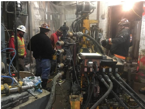
Photo 6: Drilling in Tight Corner
