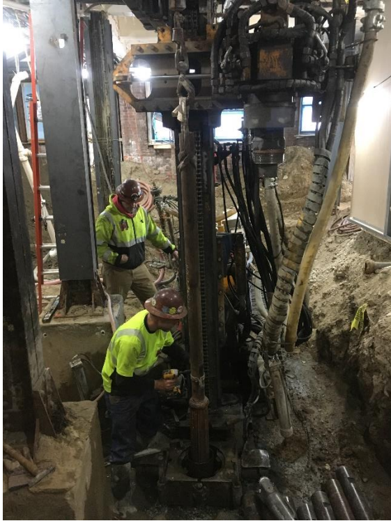
Photo 4: Drilling Next to Existing Columns
