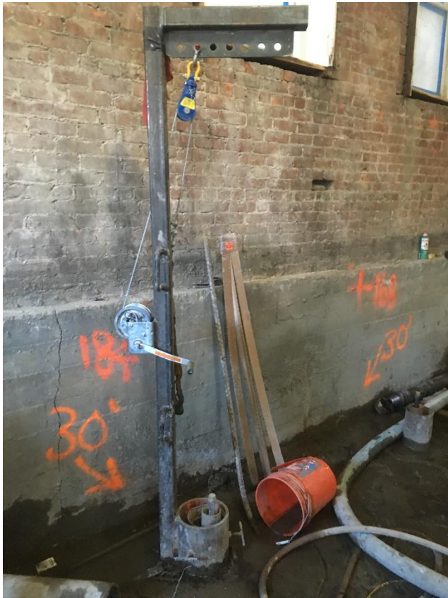
Photo 7: Hand Hoist Used to Install Expander Body
