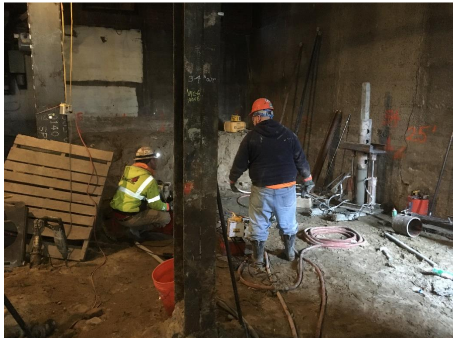
Photo 8: Hydraulic Casing Extraction Setup
