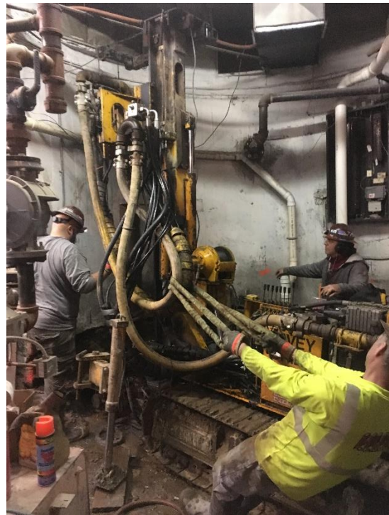
Photo 5: Drilling in the Boiler Room
